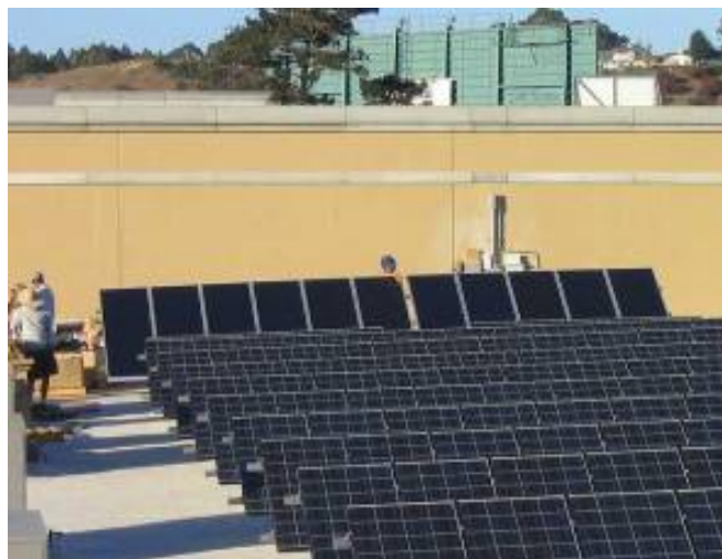
UNI-SOLAR framed modules and poly-Si modules at 30° tilt, on flat roof (SPF)
